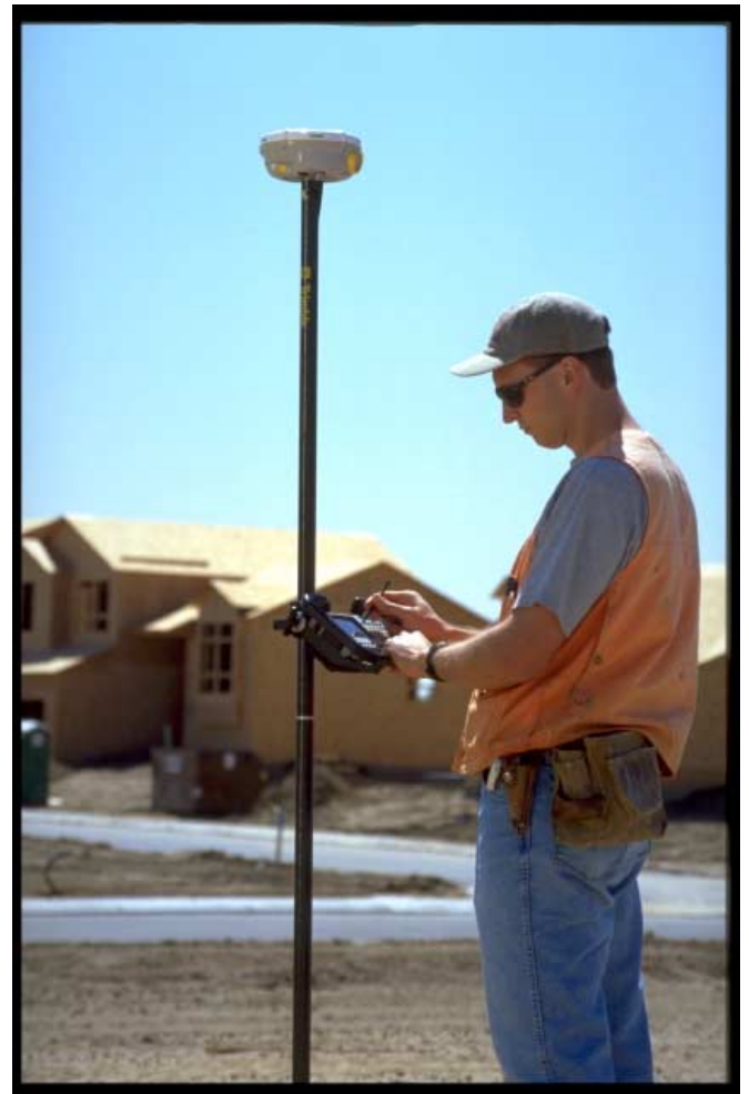
Trimble RTK all on the pole and free of cables.
